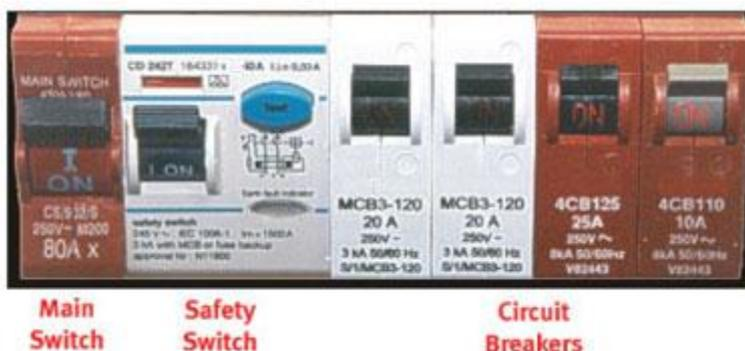
**Typical switchboard** – this shows the main switch, safety switch with test button, and four circuit breakers.
